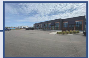
Highway commercial and retail development
